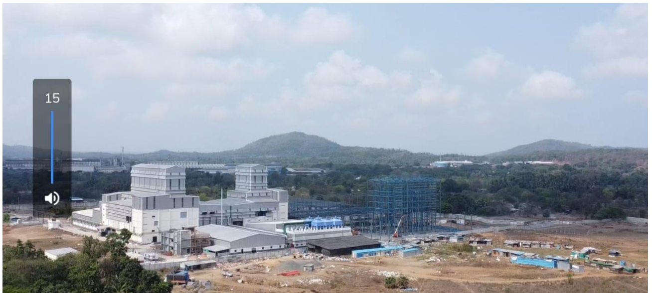
Photographs of the Carbon Black Plant under construction
